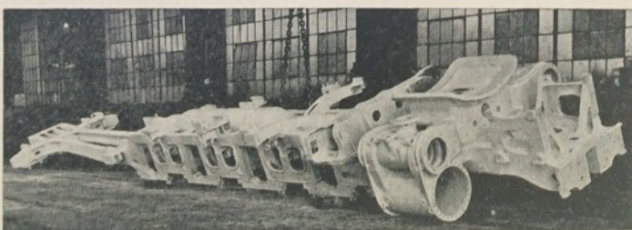
Fig. 8. Cast-steel Locomotive Beds. Above, South African Railways 2-8-4 Locomotive. Left, New York Central 4-8-4 Locomotive.
