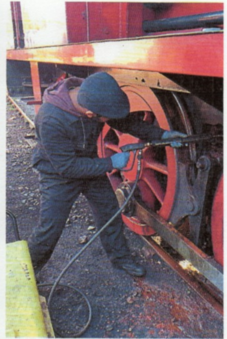
Boiler work: Muhammad washes out the boiler foundation ring, removing sludge and scale. DAVID GRINDLEY
