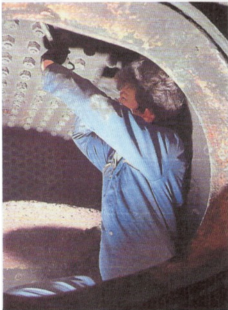
Tom provides light for a visual inspection. DAVID GRINDLEY
