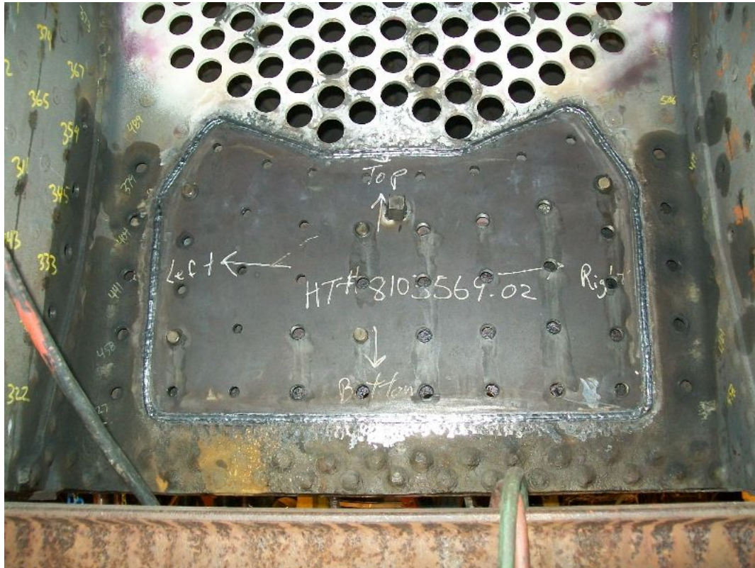
Photo of poorly designed patch repair
